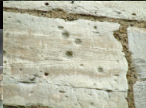
Lead projectile strikes on the limestone walls are numerous, both on the tower and the King's Manor walls. Photo Chris Rock.
