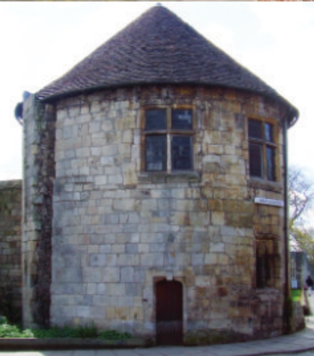
The two sections of the tower almost meet, the original medieval and the post-Civil War rebuild using reclaimed stones and added windows and doors from King's Manor. Photo Chris Rock.
